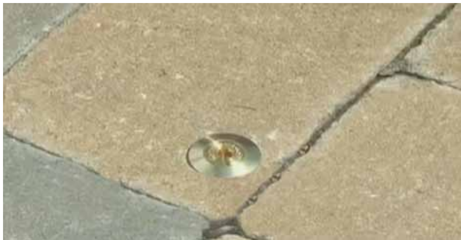
PIPE ANCHOR ASSEMBLY INSTALLED AND RECESSED WITH DECK SURFACE
