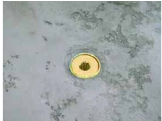
BRASS ANCHOR FLUSH WITH THE DECK SURFACE
