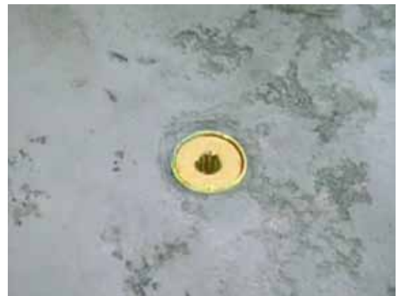
BRASS ANCHOR FLUSH WITH THE DECK SURFACE
