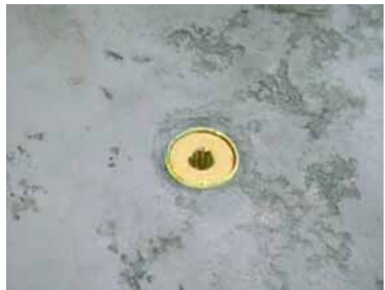
BRASS ANCHOR FLUSH WITH THE DECK SURFACE
