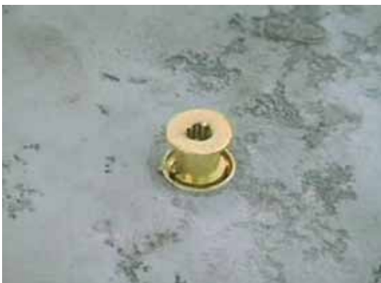
BRASS ANCHOR INSERT RAISED
