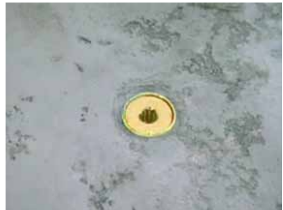
BRASS ANCHOR FLUSH WITH THE DECK SURFACE
